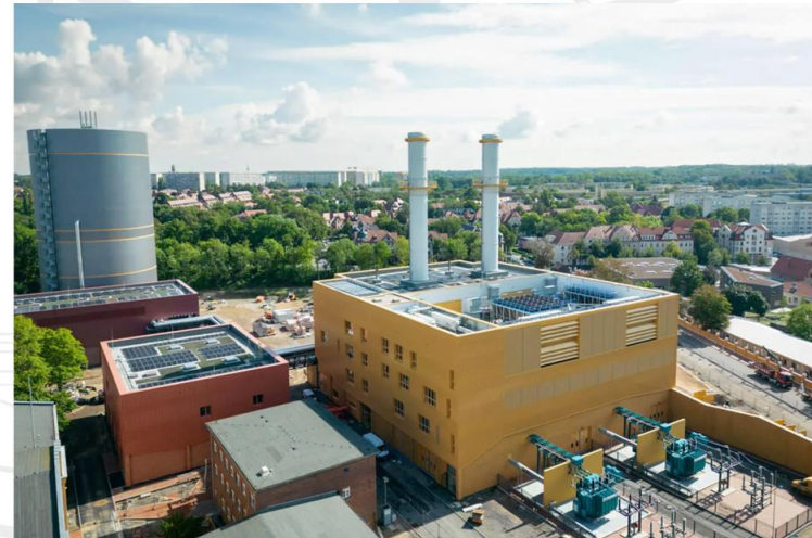
Fig. 11. Hydrogen-powered combined heat and power plant Leipzig-Süd 12 .
